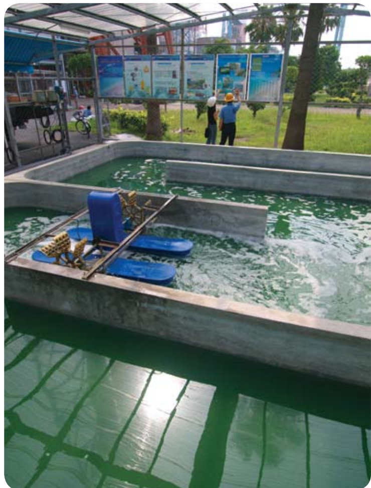
Microalgae CO 2 reduction pond in the Talin Thermal Power Plant
