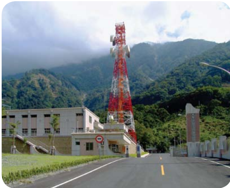
The Tachiachi Hydro Power Plant Kukuan Branch
