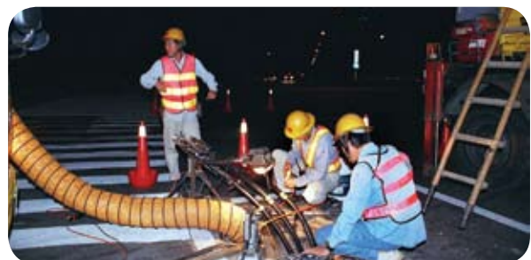
Repair and maintenance operation at night
