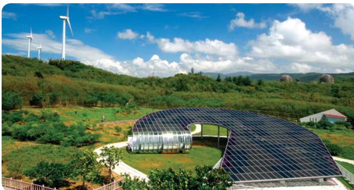
The Hengchuen solar energy pilot system
