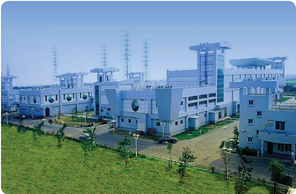
Extra high voltage (EHV) substation at the Southern Science Park
