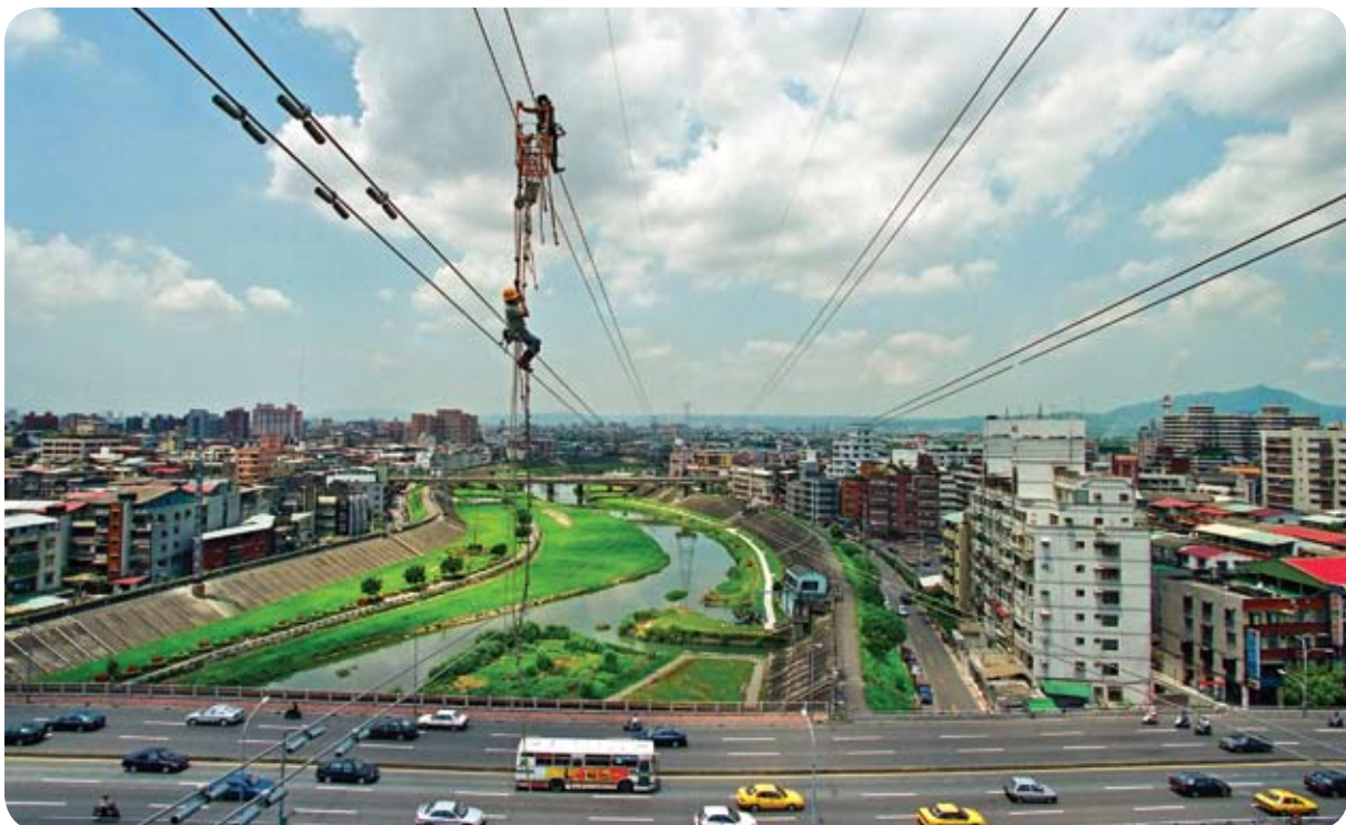
Overhead power line installation
