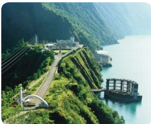
The Techi Hydro Power Plant
