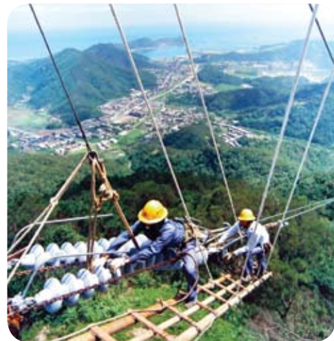
Installation of insulators in transmission lines
