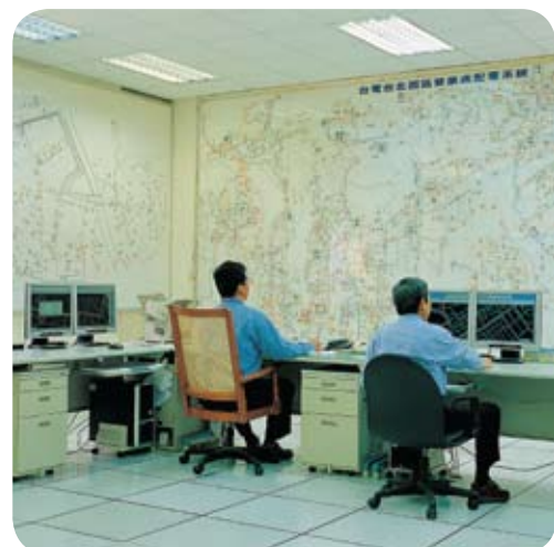
Distribution dispatching control center
