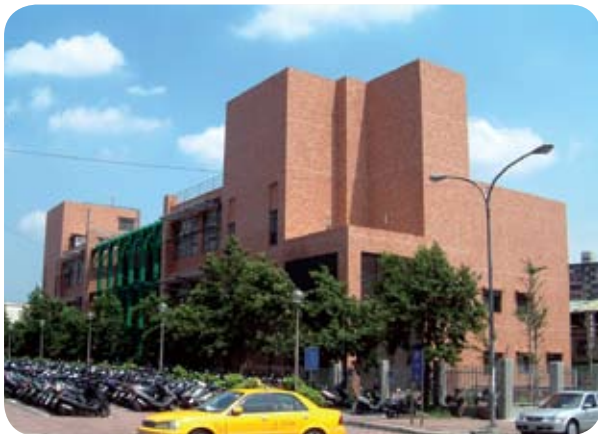
Green building – the Hsinnan Substation
