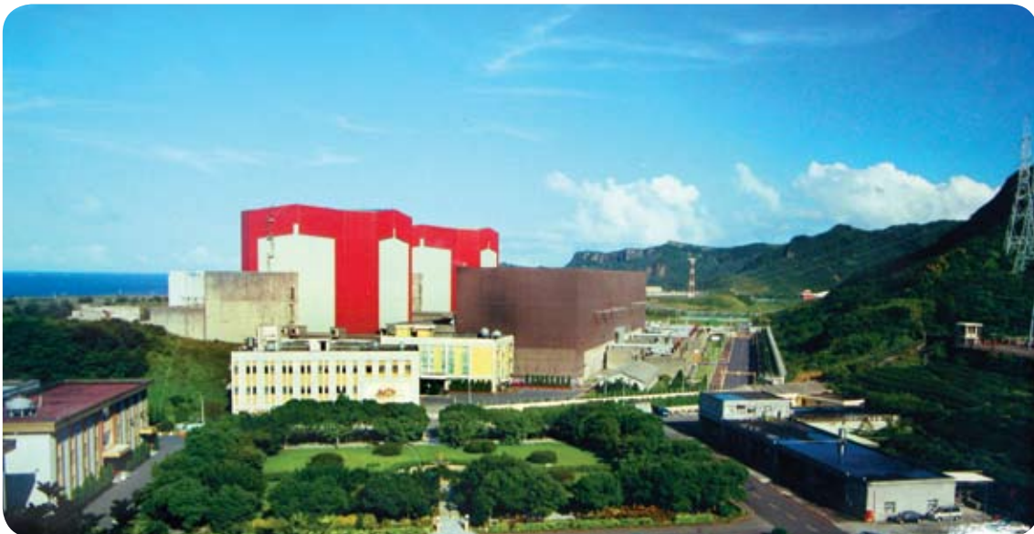
The Second Nuclear Power Plant
