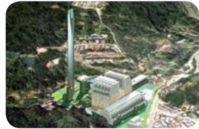
The retrofit project of the Shenao Thermal Power Plant
