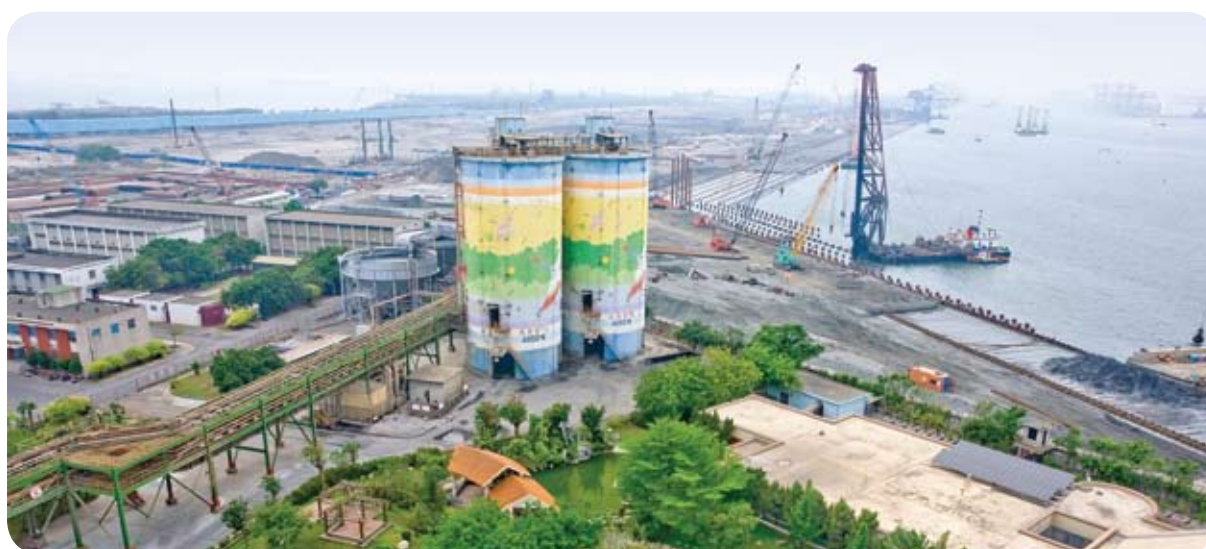
Coal ash silo facilities of the Talin Thermal Power Plant
