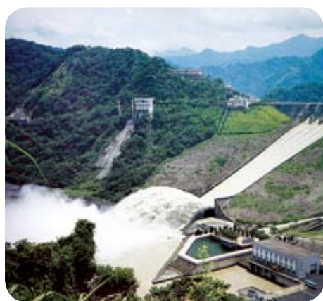
The Shihmen Hydro Power Plant
