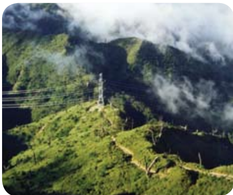
The New East-West Transmission Lines
