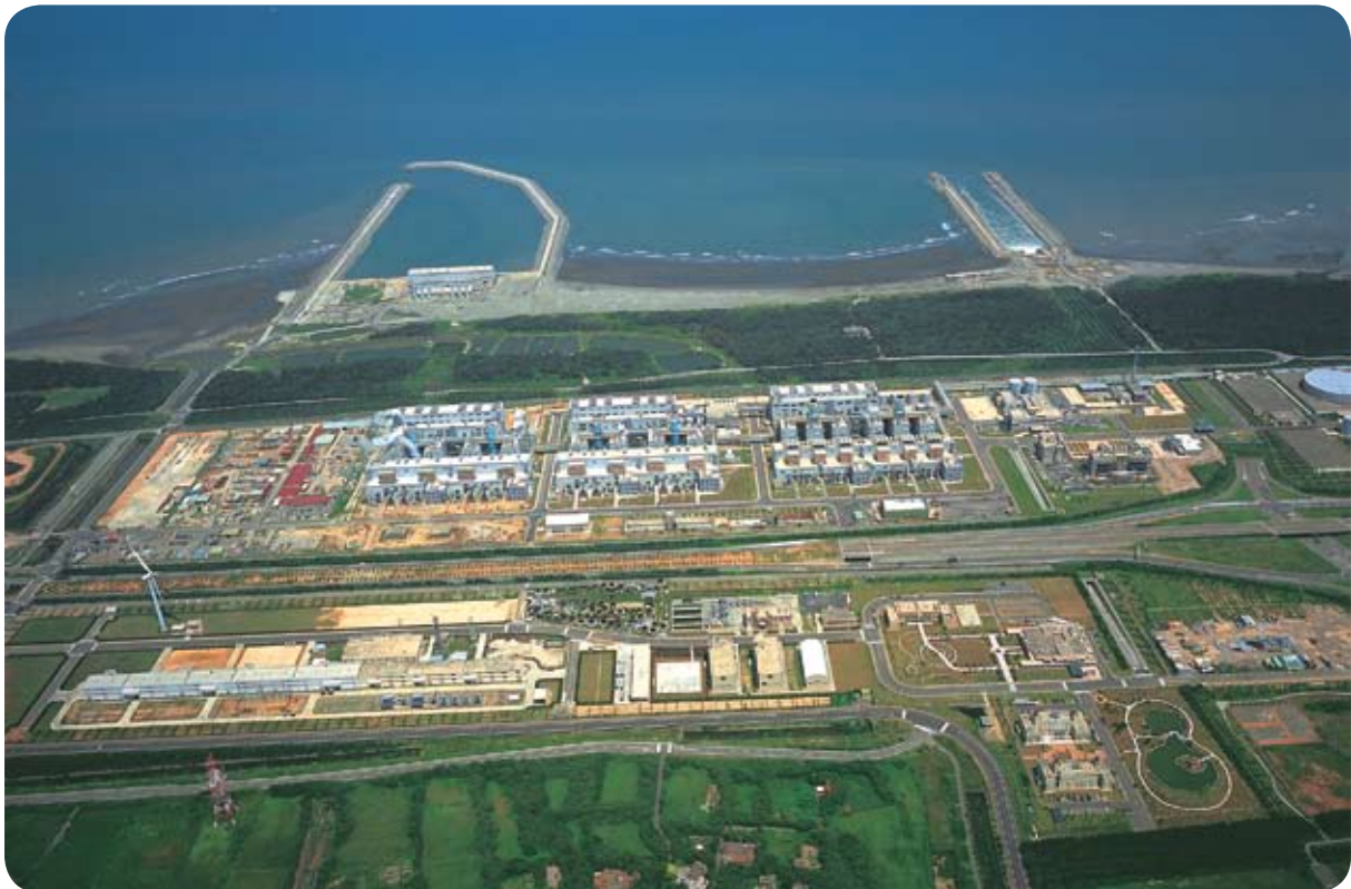
A bird's-eye view of the Tatan Thermal Power Plant
